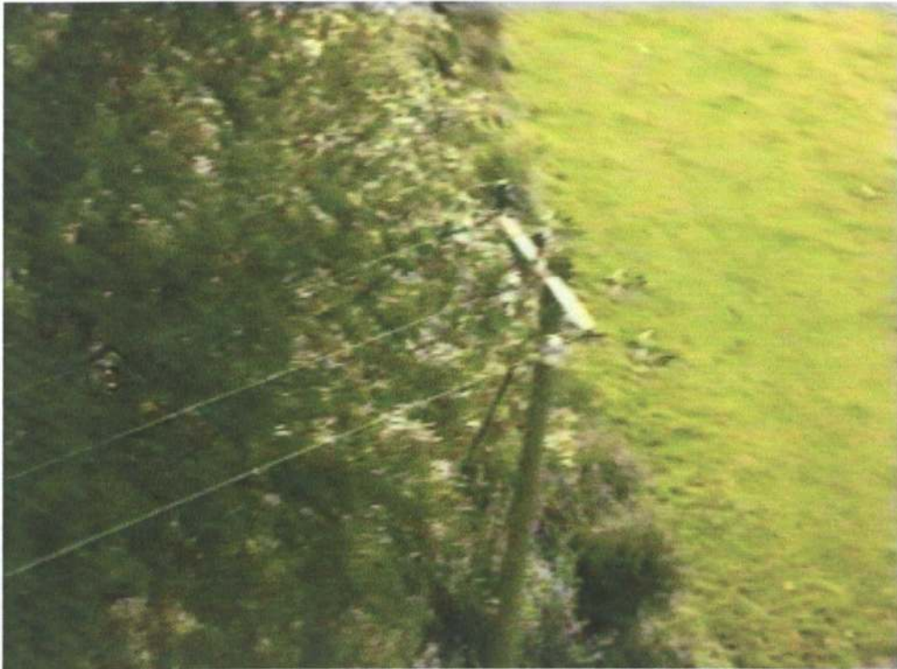
Figure 2.1: Tree Encroaching on a Power Line.
