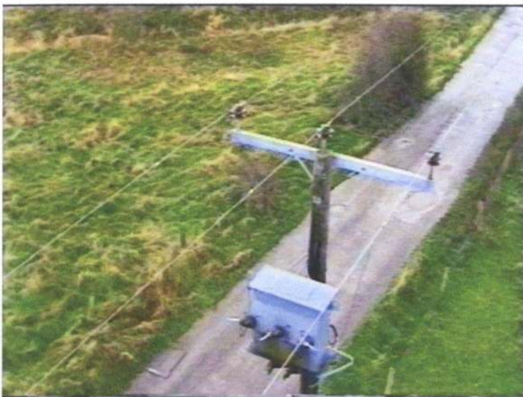
Figure 1.1: Example Support Pole showing 3-phase Conductors on Pin Insulators and a Pole-mounted Transformer.
