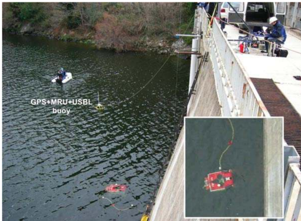
Figure 10. Experimental setup for the wall dam inspection task.
