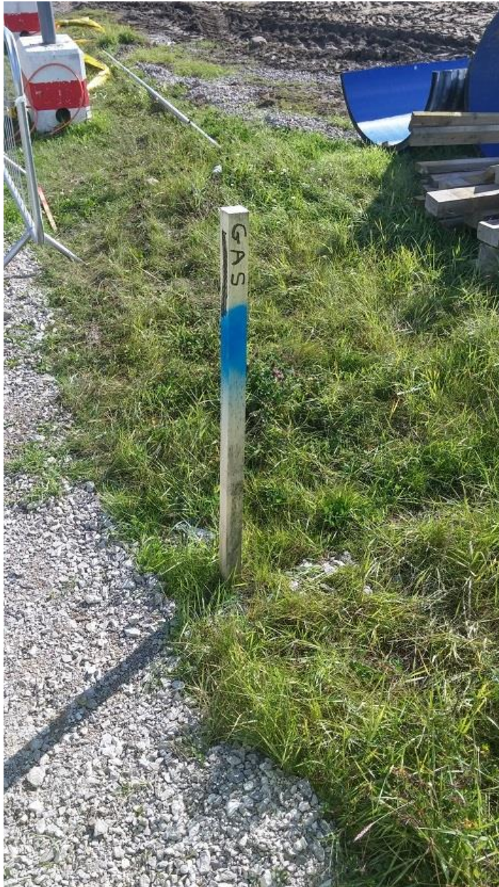
Fig 6. Marking underground utilities by using improvisational visualisation practices
