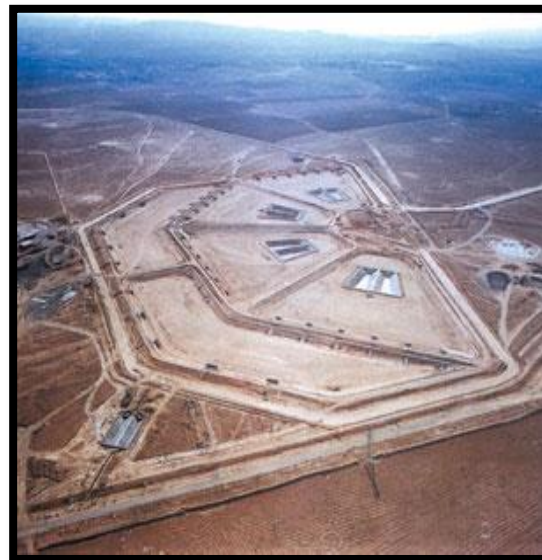
Fig.1: Overview of treatment plant
