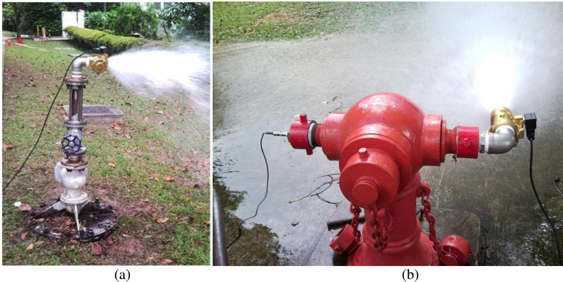
Figure 12. During leak-off experiments artificial bursts and leaks are generated by fast-opening solenoid valves connected to air valves (a) or fire hydrants (b)
