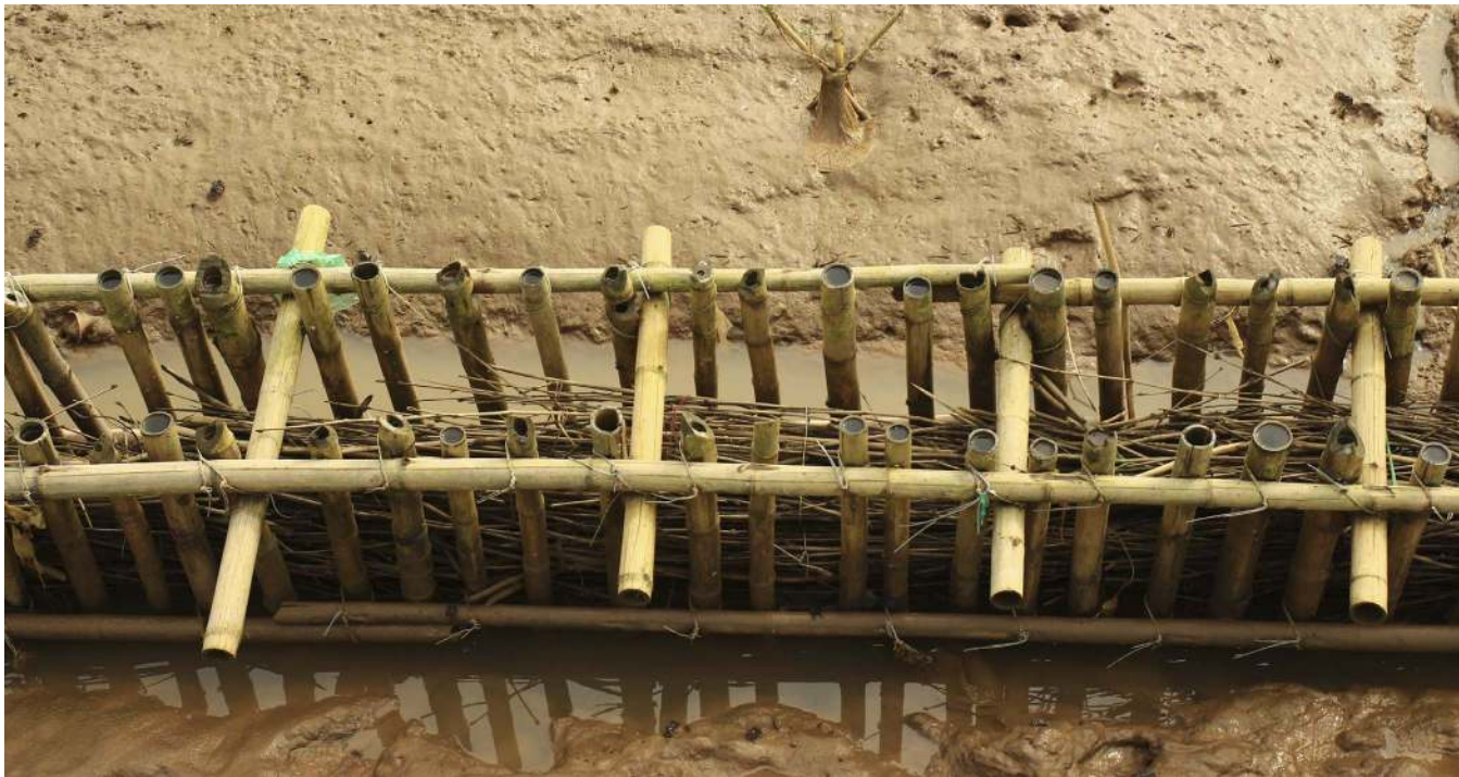
Figure 3. Fence in the field (photo by Tung Dao, 2016). The brushwood was filled to the top of the fence at the beginning but eventually washed out by waves and currents. (Color for this figure is available in the online version of this article.)
