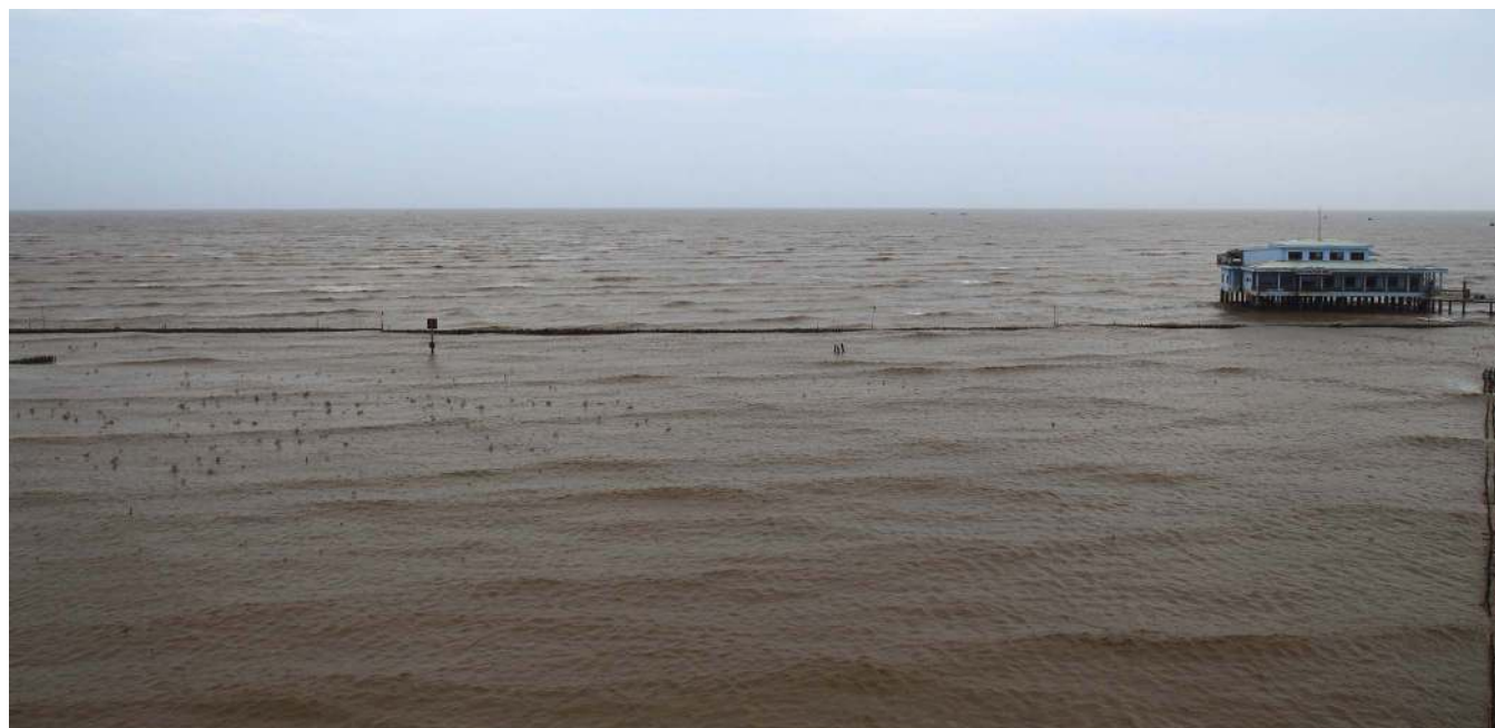
Figure 12. Wave patterns behind a wooden fence at Nha Mat in Bac Lieu Province (photo by Tung Dao, 2016). The bamboo fence is located parallel to the coast and just inshore of the building. (Color for this figure is available in the online version of this article.)
