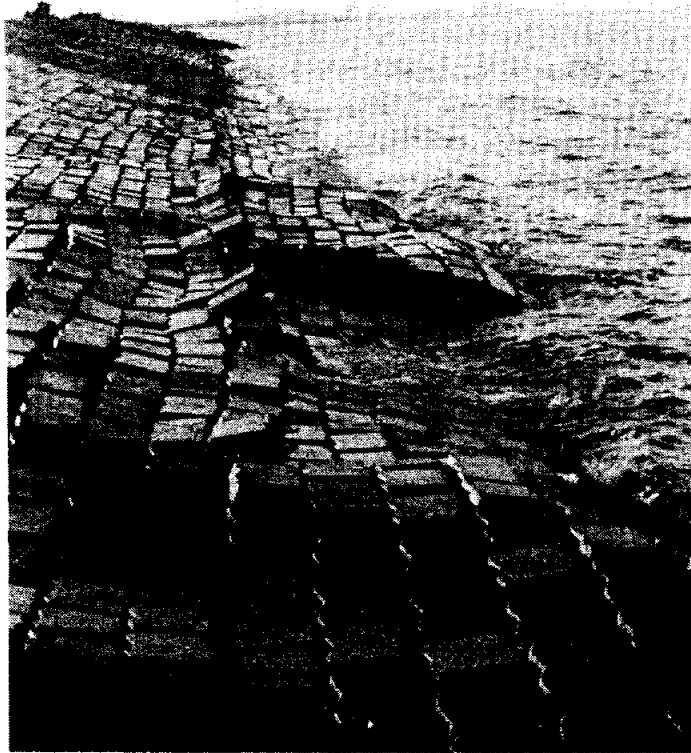
Figure 17/Photo 1. Block mattress being damaged by subsoil failure
