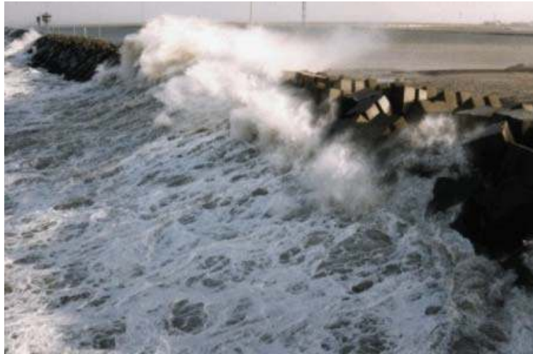
Figure 1.1: Wave run-up and overtopping at Zeebrugge breakwater during (mild) storm conditions (from OPTICREST project, www.rug.ac.be/opticrest ).
