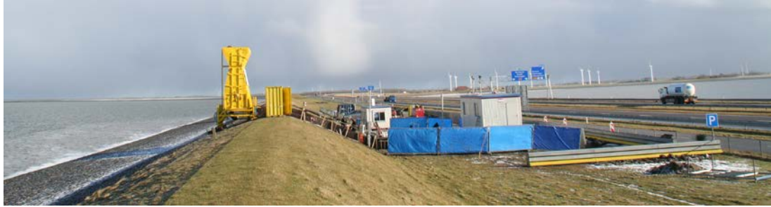
Figure 1. Set-up of the Wave Overtopping Simulator close to a highway.
