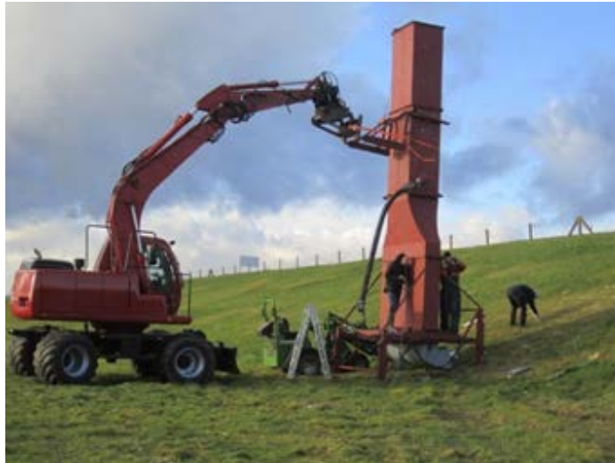
Figure 5. Calibration on a dike slope of the Wave Run-up Simulator.
