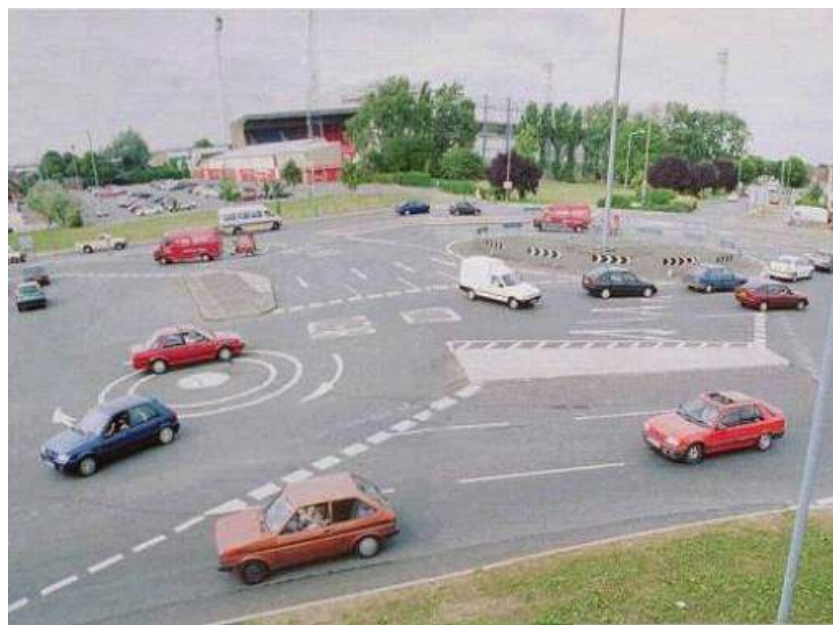
Figure 73. A photograph of the real situation of combined roundabouts.
