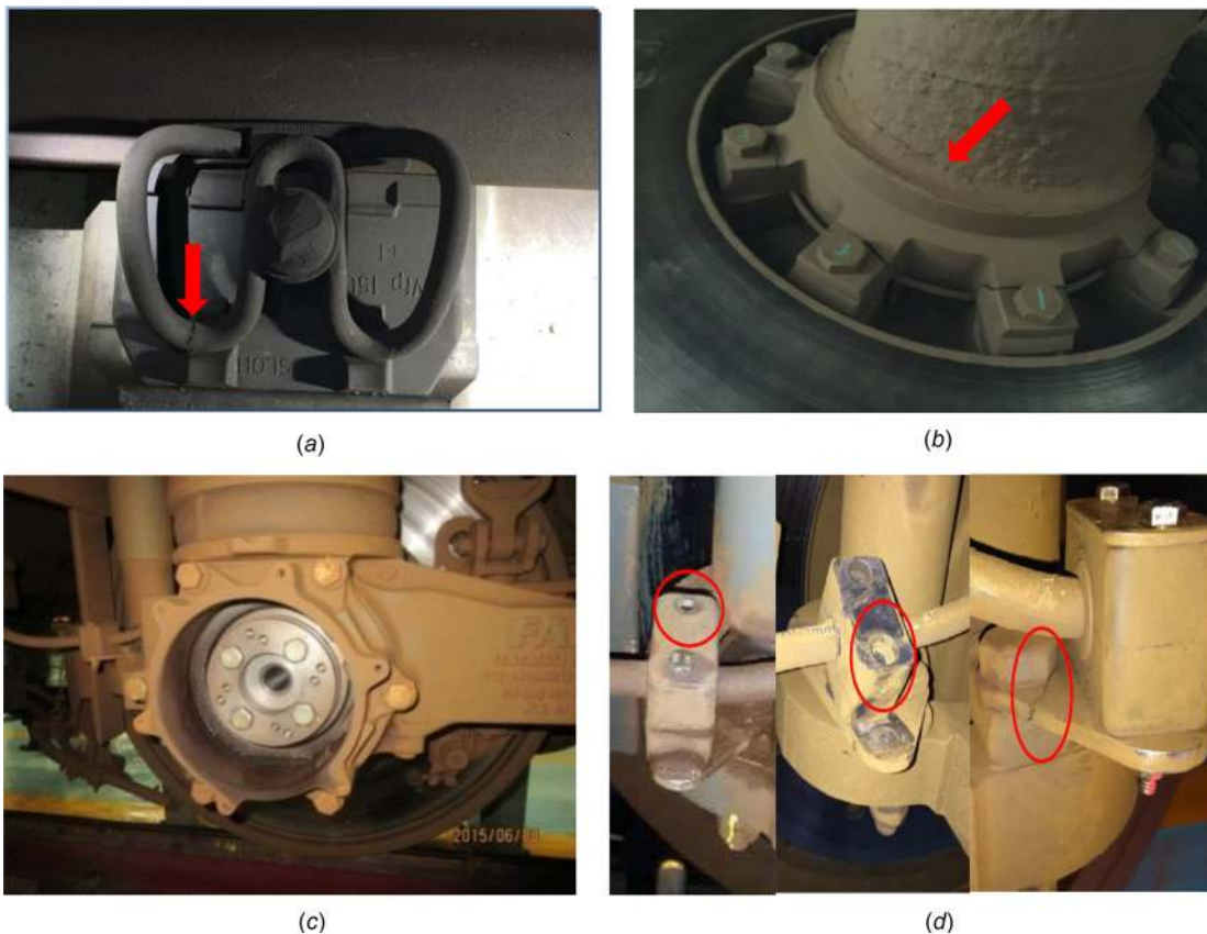
Fig. 18 Dynamic fatigue damage of vehicle and track components and accessories resulting from vibrations excited by high-order polygonization. (a) Fatigue of a clip, (b) a crack at the seat of a brake disk, (c) a missing axle box cover, and (d) missing bolts and cracks on auxiliary components of bogies.
