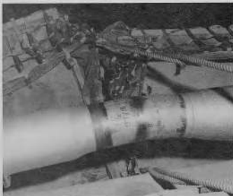
FIGURE 37 - INVAR WELD IN VJ PIPING ON A MOBILE LAUNCHER MARKED UP FOR X-RAY INSPECTION
