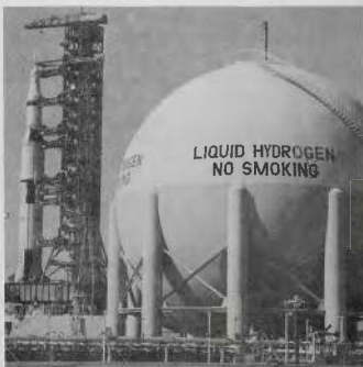
FIGURE 11 - LIQUID HYDROGEN STORAGE SPHERE
