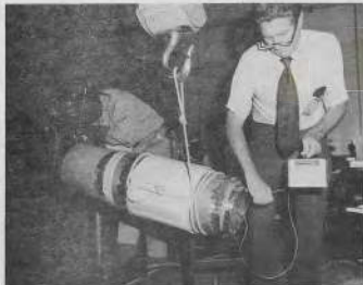
FIGURE 24 - OXYGEN ANALYZER BEING APPLIED DURING AN EARLY STAGE OF THE FABRICATION OF A VJ SPOOL PIECE
