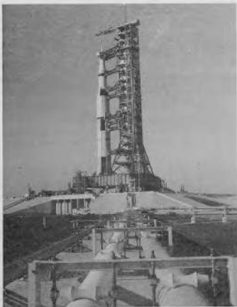
FIGURE 27 - VACUUM JACKETED PIPING INSTALLED IN A CROSS COUNTRY RUN AT A LAUNCH SITE
