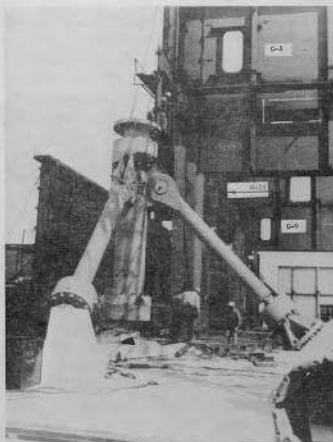
FIGURE 3 - HANGING GIRDER G-14
