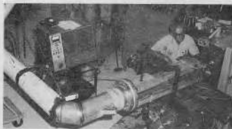
FIGURE 33 - VACUUM JACKETED SPOOL PIECE BEING HELIUM MASS SPECTROGRAPHIC LEAK TESTED DURING FINAL MACHINING IN THE LAUNCH EQUIPMENT SHOP
