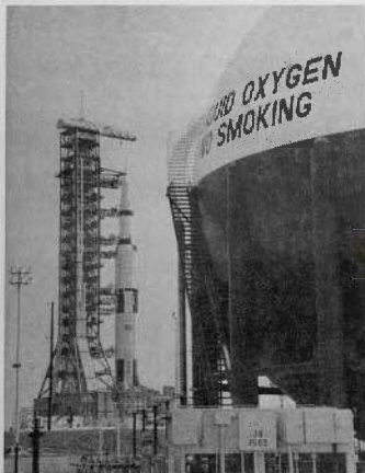
FIGURE 14 - LIQUID OXYGEN STORAGE SPHERE
