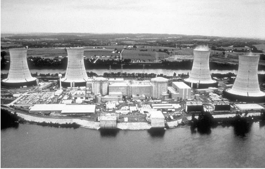
Figure 12: The nuclear power plants at Three Mile Island, Pennsylvania, USA.
