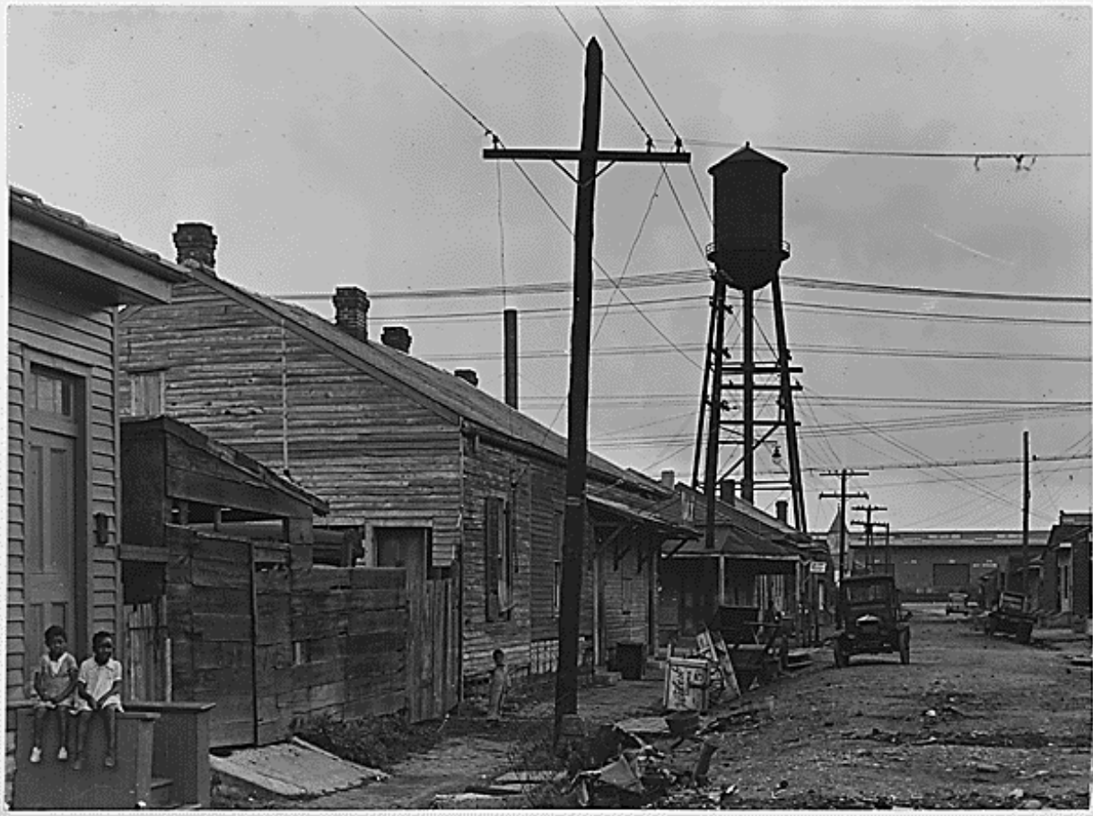
Figure 23. The St. Thomas site prior to redevelopment, circa 1940. This photograph, like many taken during this era, may have exaggerated the site's dilapidation. Source: Franklin D. Roosevelt Presidential Library.
