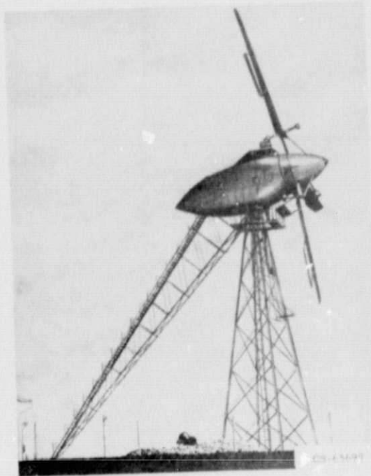
Figure 3. - 100 kW Russian Wind-Turbine.
