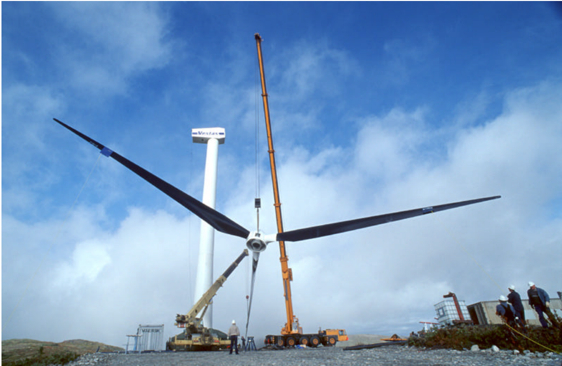
Photograph 9: the second wind turbine being installed
