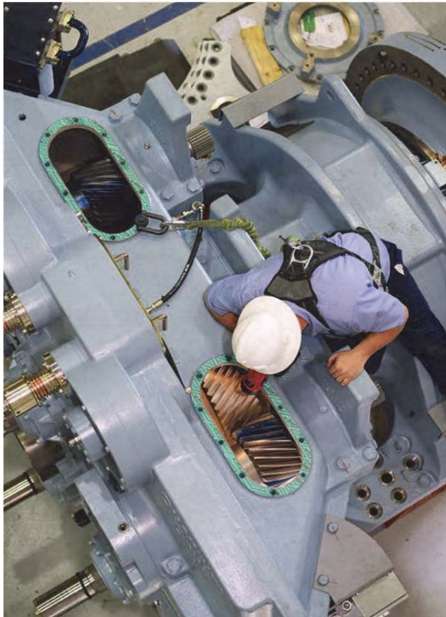
Fig. 1. Top view of a Liberty Quantum Drive 2.5 MW rated power wind turbine gearbox (Source: Clipper Windpower).
