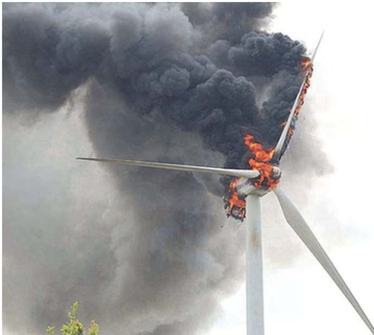
Fig. 8. A utility scale wind turbine on fire (Photo: flickr).
