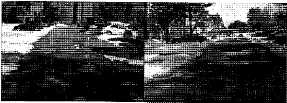
Figure 20: Pavement conditions after thawing and refreezing of meltwater (12:50PM on 2/16/08) (20a) PC at 12:50PM (left); (20b) Stnd. Ref. lot at 12:50PM (right)
