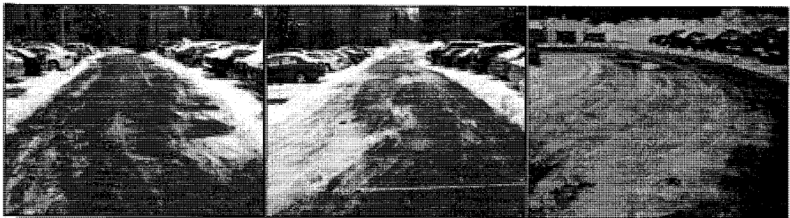
Figure 19: Pervious concrete surface conditions with varying levels of shading (11AM on 2/27/08) (19a) In sun (left); (19b) In partial sun (center); (19c) In shade (right)
