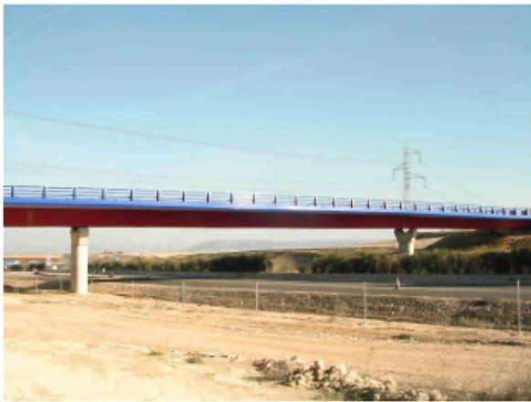
Fig. 6. Global view of the bridge.
