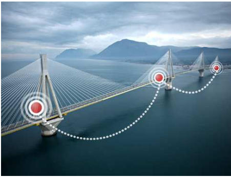
Fig. 1: wireless sensors placed on bridge [13]
