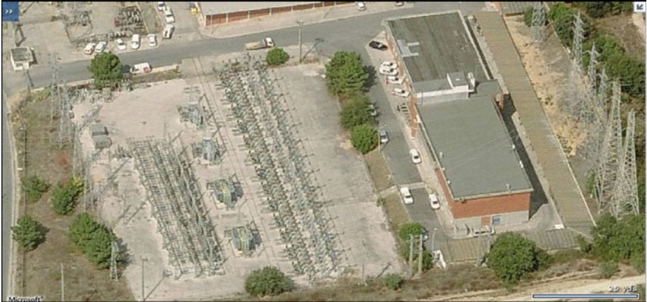
Fig. 3. Substation perimeter surveillance
