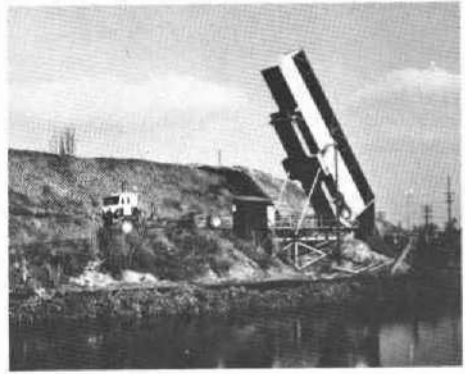
Figure 8. Unloading hogged fuel at the University of Oregon steam plant, Eugene.
