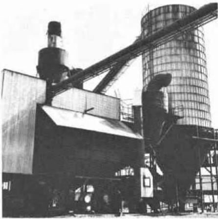
Figure 18. Automatically fired steam plant at a lumber mill in Grant's Pass, Oregon, that uses sawdust to produce steam for dry kilns.
