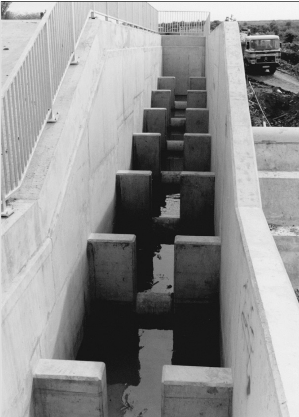
Fig. 10. Fishpass, construction near complete
