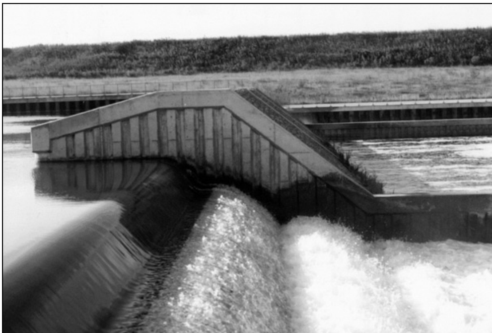
Fig. 12. Weir in operation
