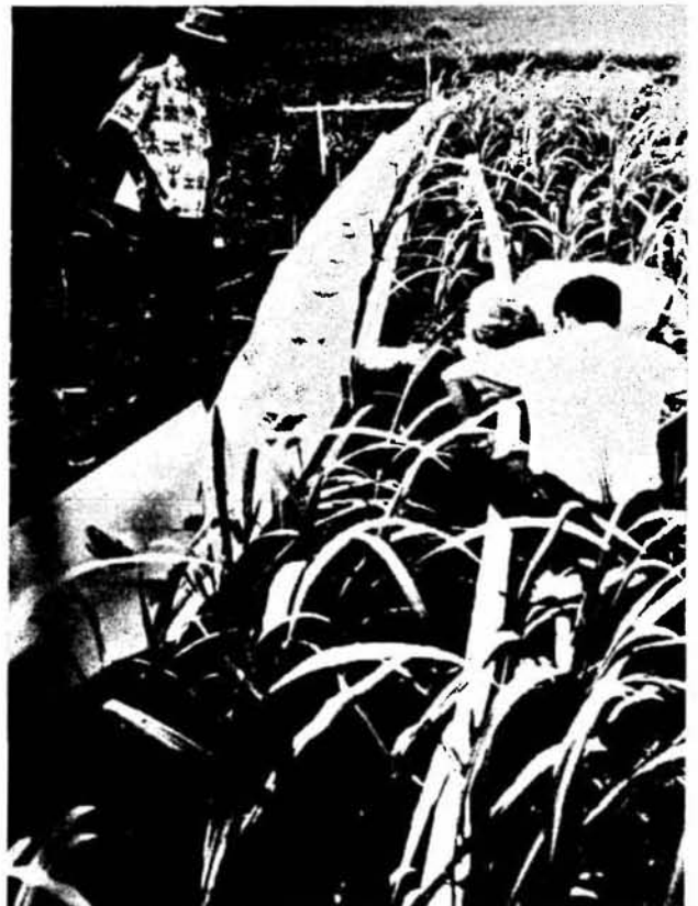
Photograph No. 4. TRANSPORT AND DISTRIBUTION SYSTEMS FOR THE IRRIGATION WATER: PVC PIPE FOR SEWAGE EFFLUENT AND ALUMINUM FLUME FOR DITCH WATER.
